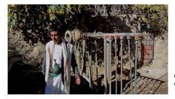
Wadi Qarada, Yemen: irrigation deep well also used for village drinking water supply (see the separate connections)
